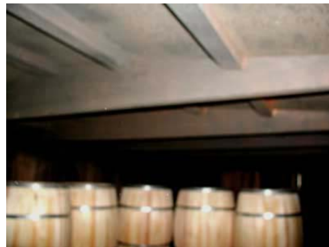
Figure 5: Interior view of the ceiling.
