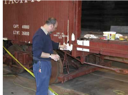
Figure 7: Wood fills being applied by the author.
